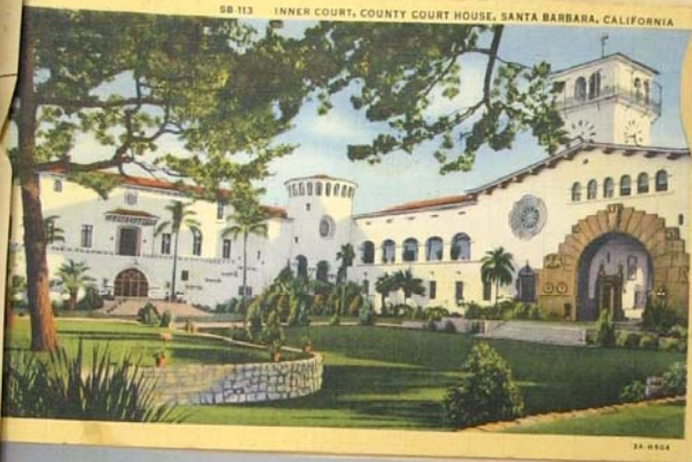
SB 113 INNER COURT, COUNTY COURT HOUSE, SANTA BARBARA, CALIFORNIA
