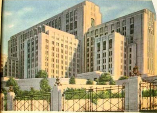
LOS ANGELES GENERAL HOSPITAL, LOS ANGELES, CALIFORNIA
