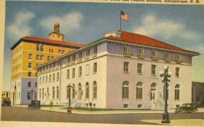
A-1 U. S. Post Office and Federal Building, Albuquerque, N. M.
